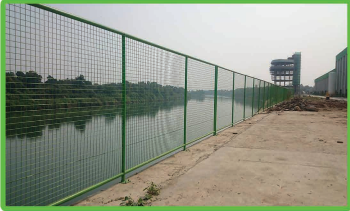
Europe & Asia Commercial (EAC) construction project
